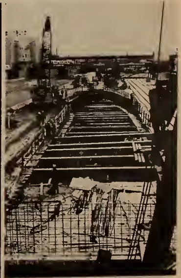
South Cove Tunnel
